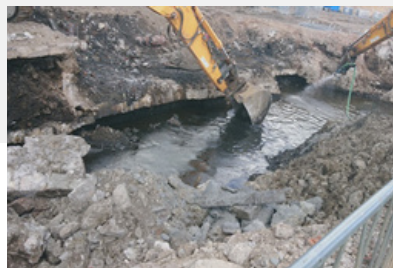
Figure 1 - Flocculant addition to hydrocarbon impacted organic sludge to dewater for handling before further ex-situ treatment.
