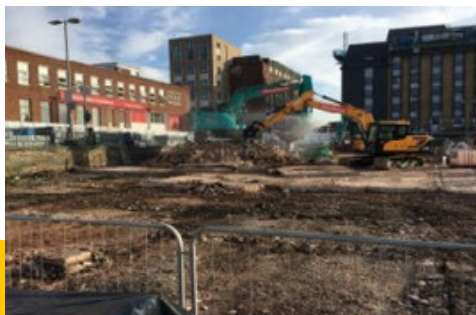
Figure 2 - Excavation of hydrocarbon impacted made ground
