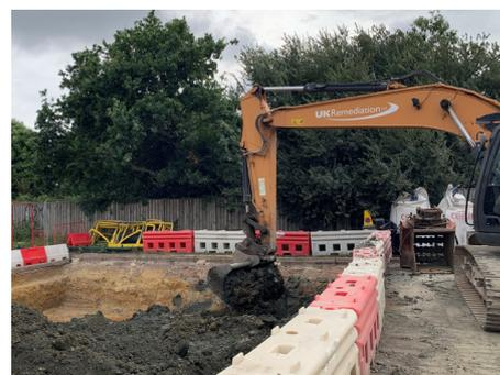
Figure 2 – Drying agent added using a specialist excavator processing bucket attachment and sealed to allow time to cure.
