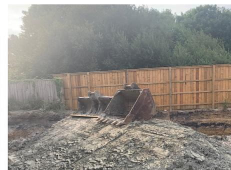
Figure 3 - Stabilised material able to bare weight post treatment and ready for disposal.
