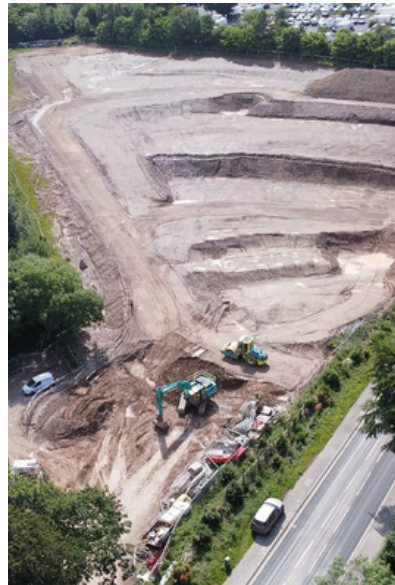
Figure 2 - Final earthworks formation levels
