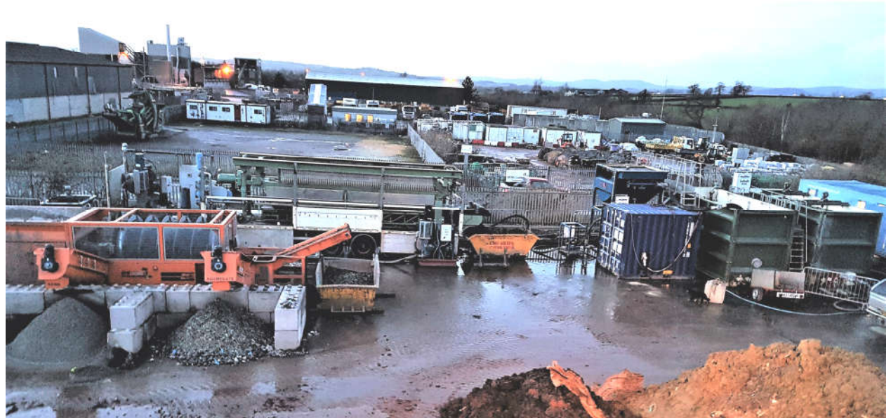
UK Remediation soil washing train deployed at our facility near Exeter.
