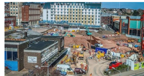
Busy city centre site: Remediation works visible at rear
