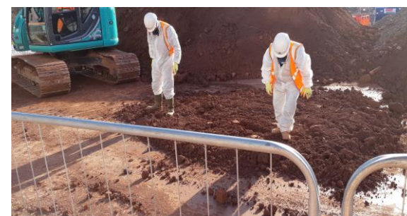
Small batch picking of asbestos within the controlled area
