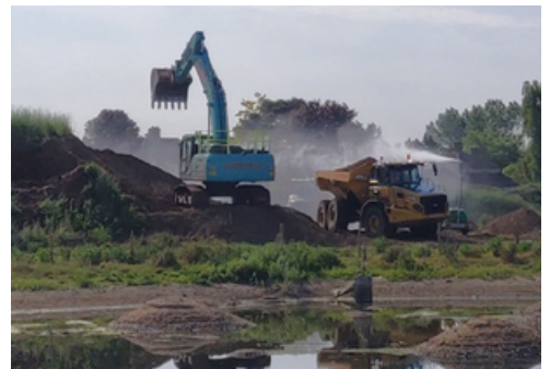
Dust suppression applied whilst working close to a nature conservation area.
