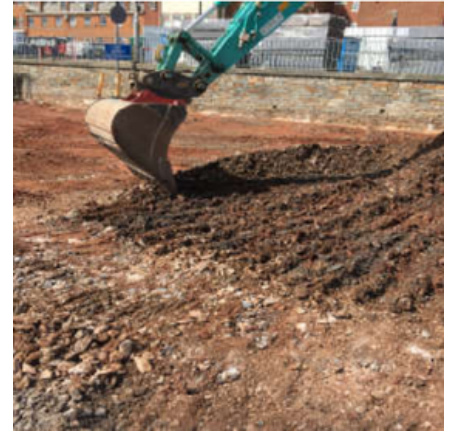
Figure 2 - Excavation of hydrocarbon impacted made ground
