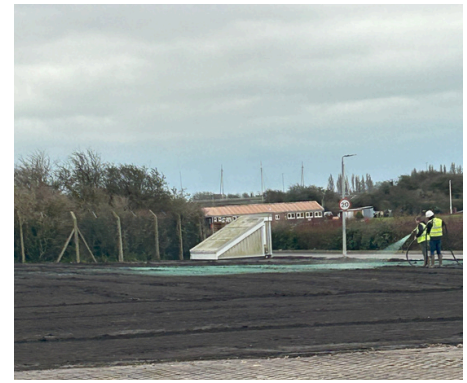
Hydroseeding in progress (green dye shows where applied)
