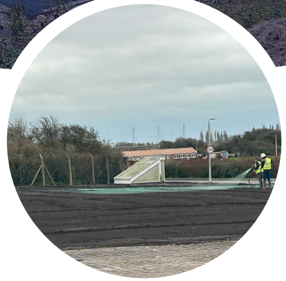
Hydroseeding in progress (green dye shows where applied)
