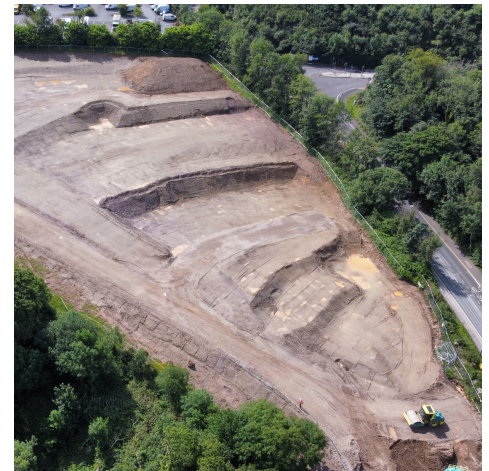
Figure 2 - Final earthworks formation levels.
